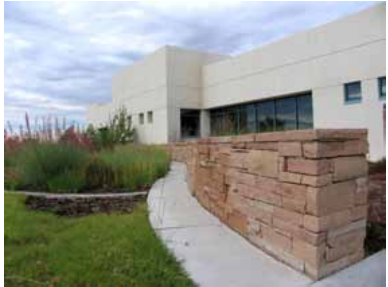
Newer business incubators are found on college campuses and research parks. While some incubators are in older modified buildings, many communities are investing in state-of-the-art facilities, such as the Quality Center for Business in Farmington, NM.
